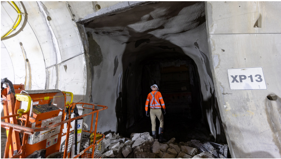
Cross passage excavation.
