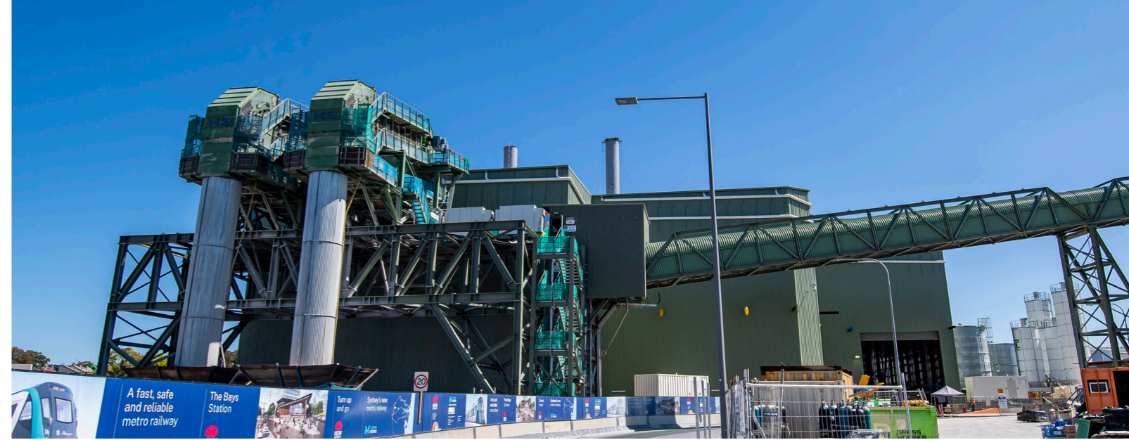
Vertical conveyors at The Bays Station site.
